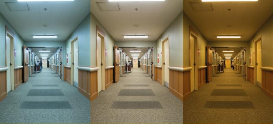
The new tunable LED lighting in the ACC Care Center corridor, shown at the morning setting (specified as 6500K at 66% output, left), the afternoon setting (specified as 4000K at 66% output, center), and the nighttime setting (specified as 2700K at 20% output, right). Photo: Sacramento Municipal Utility District
